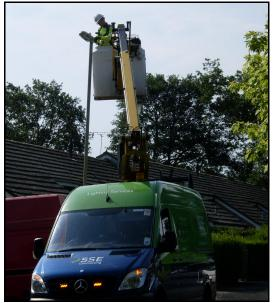
more concentrated light. The picture here shows Southern Electric Contracting connecting up a newly-installed lamp post in the Burney Bit.
